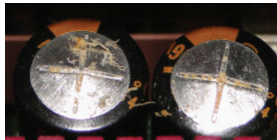
Figure 2 - Domed, Leaking Capacitors
